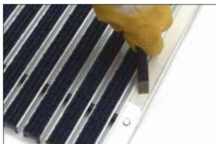
2. Please note: Dirt, ribbed carpet and glue must be removed from the aluminium profile (e.g. using a chisel).
